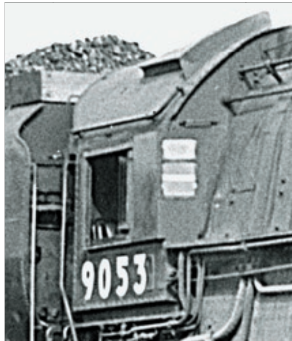
The image to the left shows the final post-war cab configuration with enlarged and relocated cab with extended cab side windows and modified front windows. Also notice the sunken footboards below the road number.
